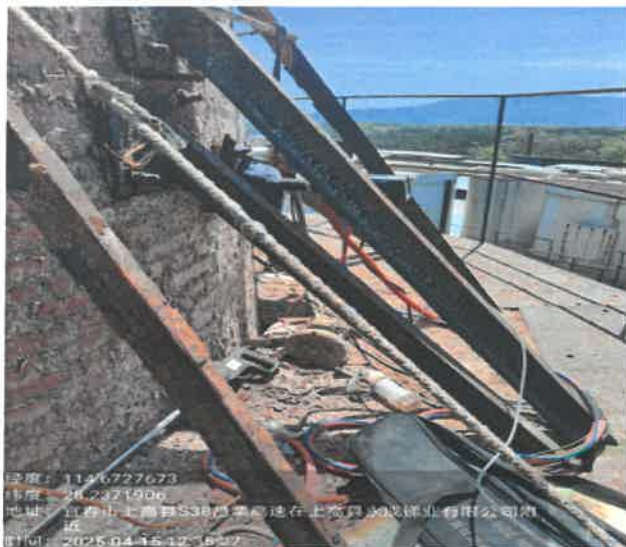
G1 废气排放口 DA001
