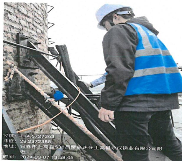
G1 废气排放口 DA001
